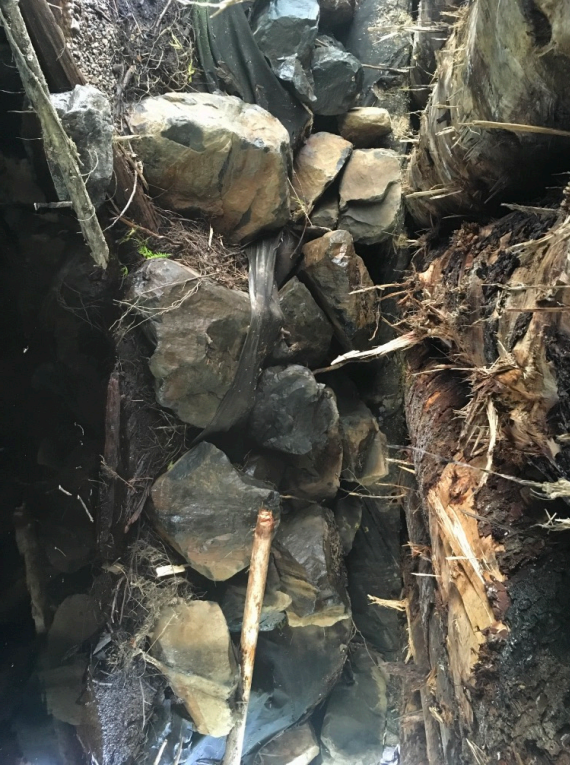
Left Bank Abutment when facing downstream
